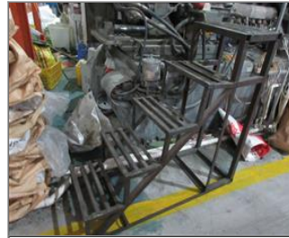
Photo of non-conformity NC-ladder without handrail.JPG
