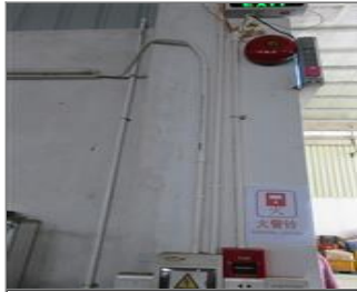
Photo of fire safety equipment Fire alarm.JPG
