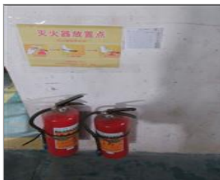
Photo of fire safety equipment Fire extinguisher.JPG
