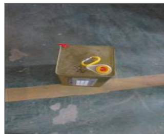
Photo of non-conformity NC-one barrel of glue without secondary container.JPG
